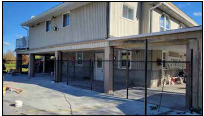
Oct. 28 - Fencing being installed
