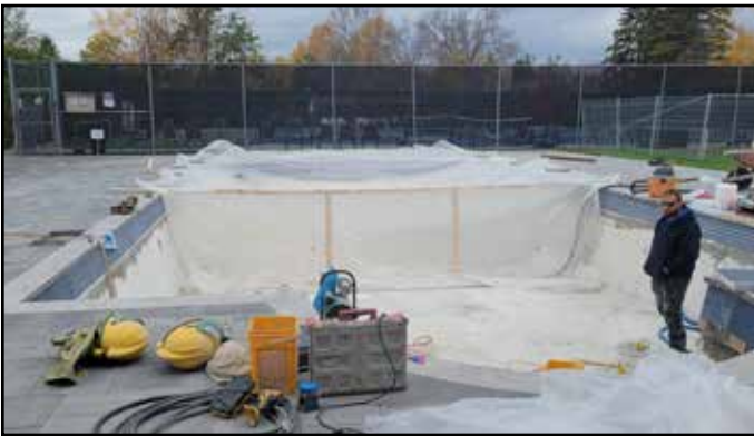
Oct. 25 - Stonework almost finished, tile getting grouted
