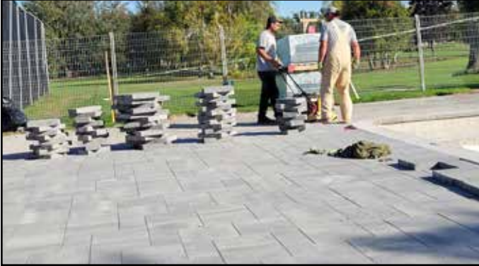
Oct. 1 - Stonework going down on the new pool deck
