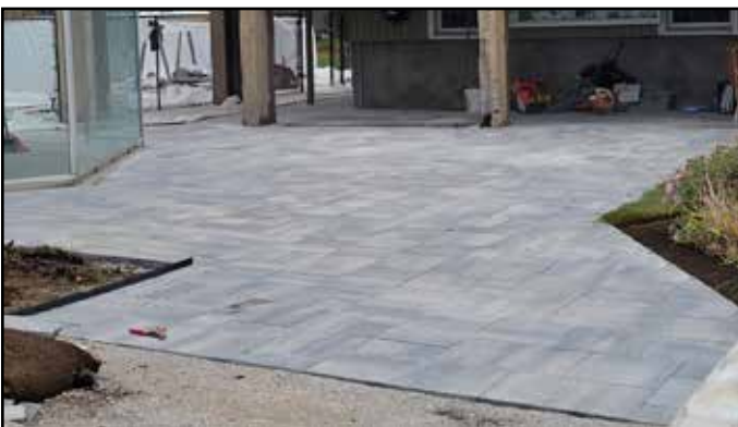
Oct. 25 - Stonework extended to kiosk area and front walkway
