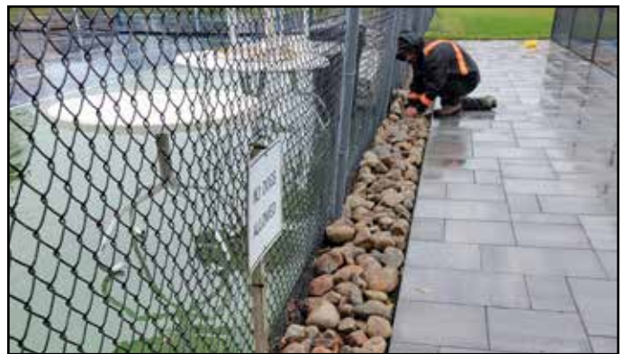
Oct. 30 - Finishing touches with river rock
