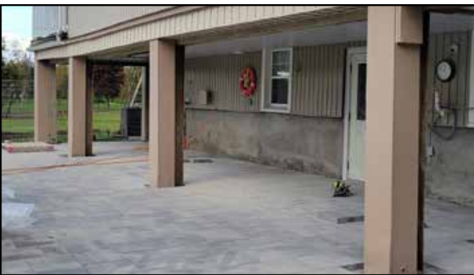
Oct. 25 - Stonework extended to building
