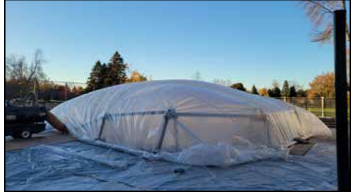
Oct. 27 - Tiling and grout covered to cure
