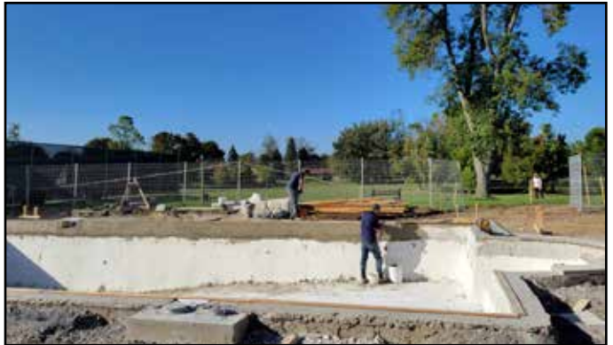
September 17 - Coping starting to go on and prepping for tiles
